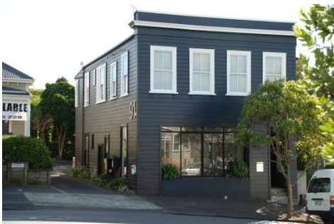
William Aitken & Co. Freeman's Bay Auckland Office. Built in 1885.
